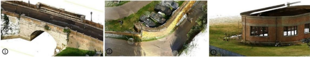
Fig. 5- Point cloud details: 1) bridge and eastern curtain wall; 2) bastion orillon, via Morandi; 3) building on the SE bastion orillon (graphic elaboration by Gianlorenzo Dellabartola, 2025)
