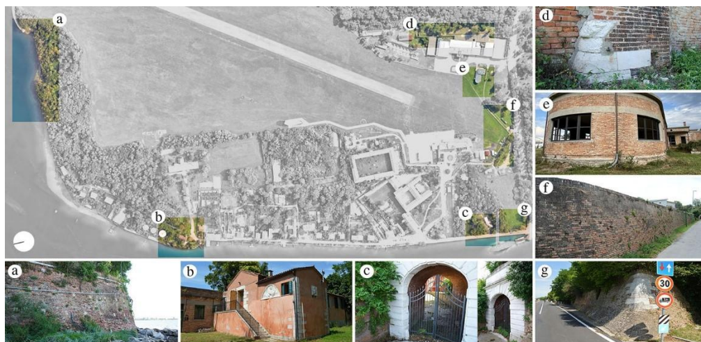
Fig. 2- Surviving fortress elements: a) Northern curtain wall; b) Castel Vecchio; c) Austrian portal; d) SE trincea corner; e) SW orillon; f) SW traversa ; g) SW lagoon-facing corner (photos by the authors, 2025)
